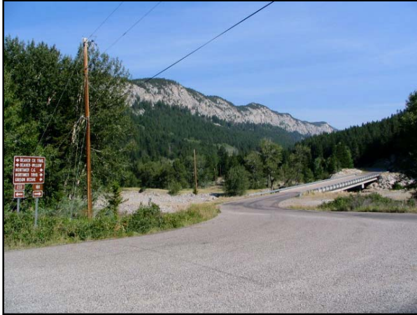
FIGURE 5. Typical layout of FDR 108 east of Gibson Dam near Blacktail Gulch Bridge.
